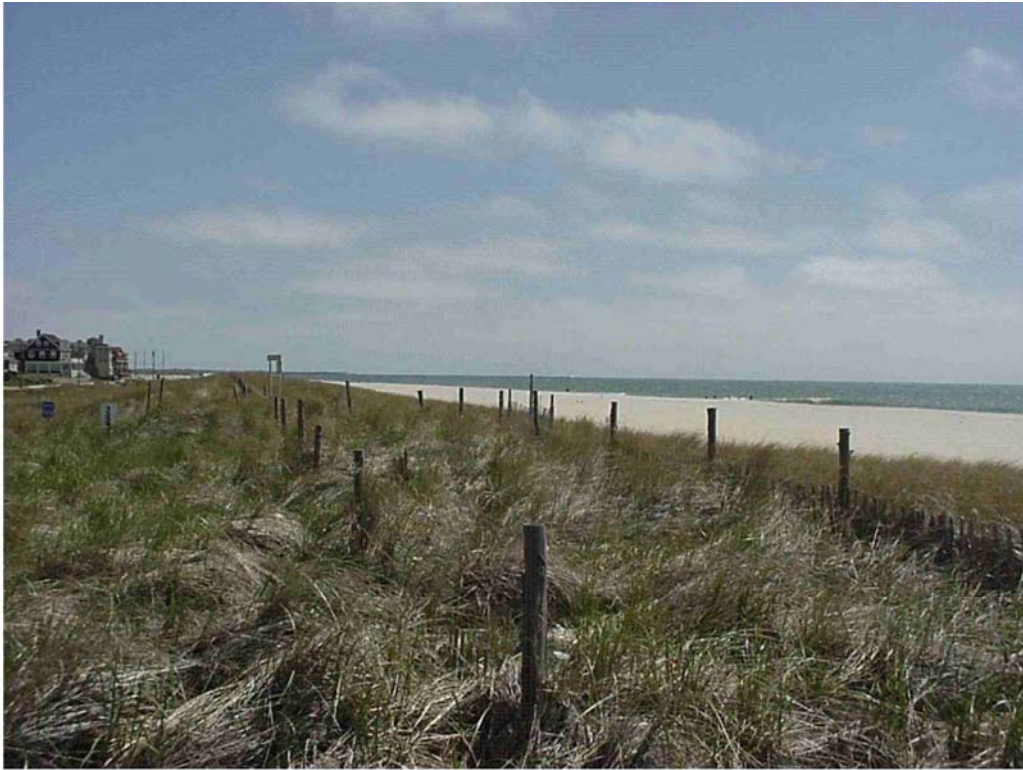
Photoplate 8a. Picture taken May 7, 2001 shows the developed berm and densely vegetated dune following 10 years of Federal beach restoration project management. Three lines of snow fence are buried and the beach remains wide for recreational purposes at Baltimore Avenue, Cape May City.
