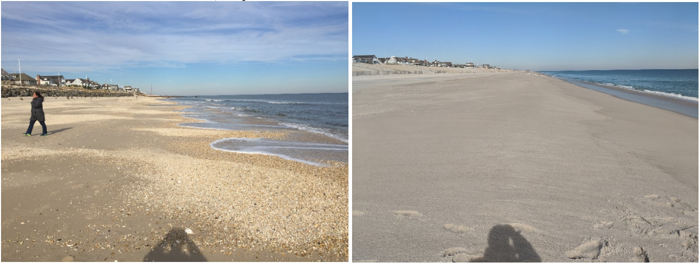
Prior to the beach fill, the Johnson Avenue profile consisted of no dune, exposed rock revetment, and a narrow beach (left photo taken December 19, 2018). The right photo (taken November 15, 2019) shows the dune (covering the rock revetment) and berm conditions five months after project completion. The position of the 0.0 ft NAVD shoreline moved seaward (205.5 ft) between surveys 57 and 59.
