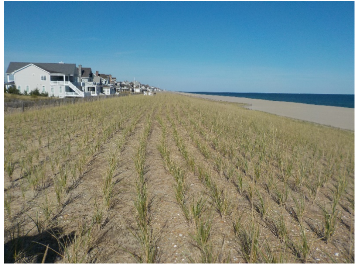
The vegetated dune at 1117 Ocean Ave. in Mantoloking covers a steel bulkhead that was constructed in 2015 (left photo taken December 19, 2018 following beach fill). The right photo (taken November 4, 2019) shows the condition of the dune vegetation and berm width similar to 2018. The 0.0 ft NAVD shoreline moved landward (-7.75 ft) from its fall 2018 position.
