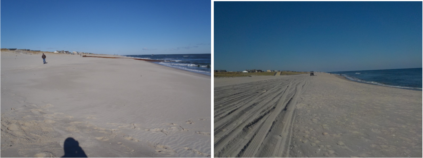
The photos of the 6 th Lane location (left December 18, 2018 and right taken November 5, 2019) show changes of the berm before and after the beachfill which was completed in February 2019. The shoreline was moved 95.75 ft during this timeframe.
