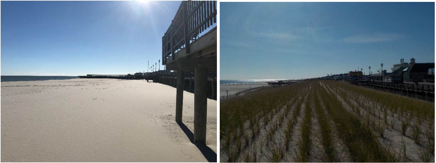
The berm and dune at the Franklin Avenue site changed significantly due to the beachfill activities that finished in January 2019 (left photo taken December 18, 2018 and right taken November 6, 2019). After years of no dune protection, the federal project included an engineered dune adjacent to the boardwalk.
