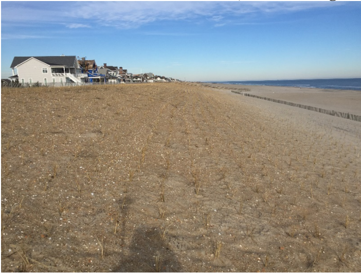
The vegetated dune at 1117 Ocean Ave. in Mantoloking covers a steel bulkhead that was constructed in 2015 (left photo taken December 19, 2018 following beach fill). The right photo (taken November 4, 2019) shows the condition of the dune vegetation and berm width similar to 2018. The 0.0 ft NAVD shoreline moved landward (-7.75 ft) from its fall 2018 position.
