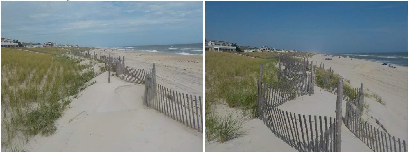
Since fall 2018, sand fencing continued to trap windblown sand at the dune toe at this Beach Haven profile location (left taken September 17, 2018 and right taken September 11, 2019). The sand accumulation reached an elevation of 14 ft NAVD88.
