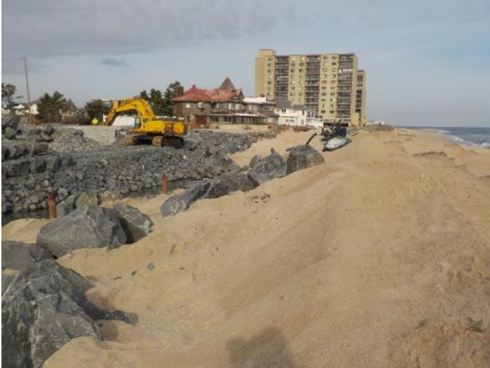
The left photo taken January 2, 2019 and shows the extensive seawall construction going on at the site establishing the rock barrier to the interior. As of December 23, 2019 the rock wall was complete and the sand pipeline was in place on the beach.
