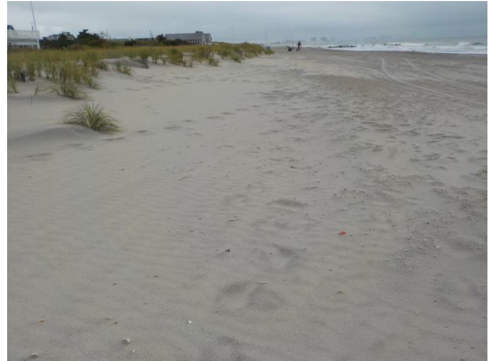
Figure 453a & 453b. The Gardens Road site is the northernmost profile in Ocean City and located in proximity Great Egg Inlet. (Left photo is from September 1, 2015. Right photo is from September 20, 2016). The dune and some of the berm that was created by the 2013 Federal emergency beach fill remained throughout 2015 and 2016. Seasonal berm elevation changes occurred, but the shoreline position was relatively constant. Over the 18-month study interval the site saw 25.21 yds 3 /ft in sand volume gains combined with a 28 ft shoreline advance.
