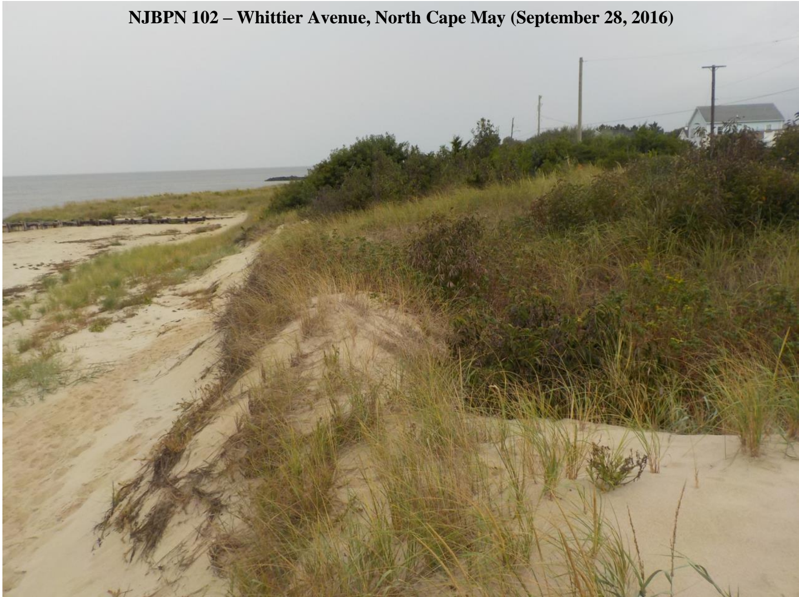
Figure 620. This view to the north along the Delaware Bay shoreline shows the massive dune developed above the seaward edge of the Cape May bluff at this site, along with the smaller hard structures (groins) put in to slow sand transport. The dune and beach system is substantial for the bayshore and remains relatively stable.
