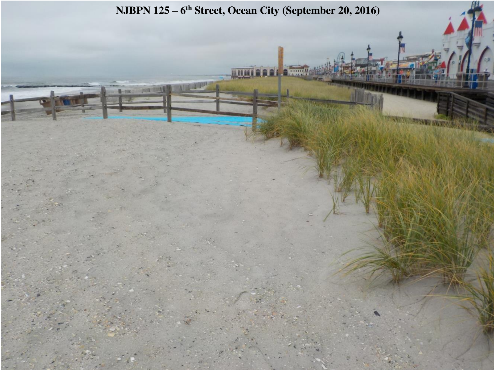
Figure 458. Sixth Avenue in Ocean City is subject to rapid rates of erosion. This view to the south shows the dune toe near the boardwalk and the existing berm at the beach. The pedestrian access path is at the end of 6 th Ave.
