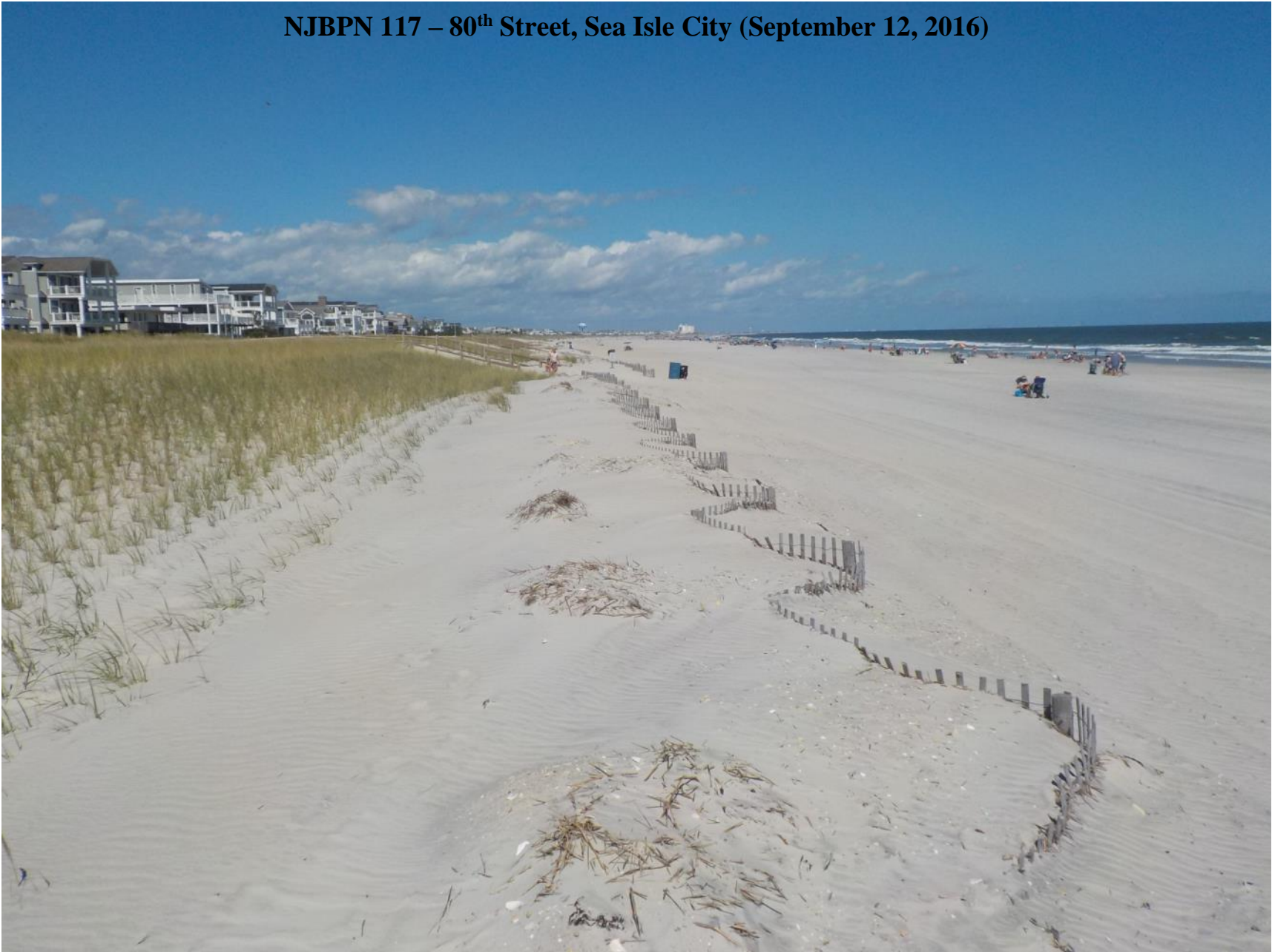
Figure 518. View to the north along the dune toe at the south end of Ludlam Island. The fencing was all but buried within a year of its installation.
