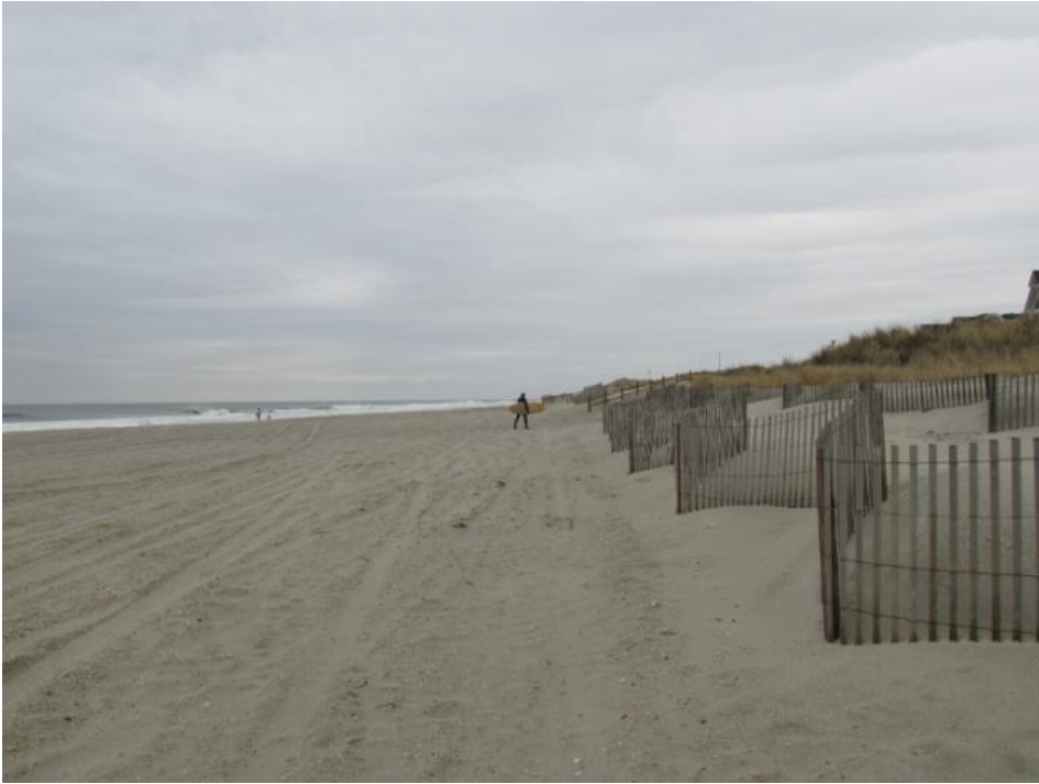
Figure 525a & 525b. The 9 th Street site is located near the Townsend's Inlet south jetty. The left photo taken, on October 7, 2015, followed an Avalon-funded beach restoration in 2015 augmenting the post-Sandy federal work in 2013. Sand filled in the fencing nearly to the top of the 4-foot fence, but shoreline retreat due to several storms and frequent onshore wind and wave conditions was so extensive, that by September 8, 2016, the beach was at the 12 th Street revetment rocks three blocks south of the site.
