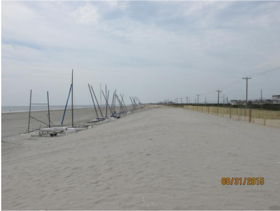
Figure 501a & 501b. Photo on the left was taken August 31, 2015 at the toe of the new foredune and the original dune that is located landward of the new fence was constructed in 1998 with a geo-tube core. The photo on the right was taken September 13, 2016, which was a year after the federal project. The dry beach width was increased and aeolian transport resulted in sand accumulating on the seaward dune slope.
