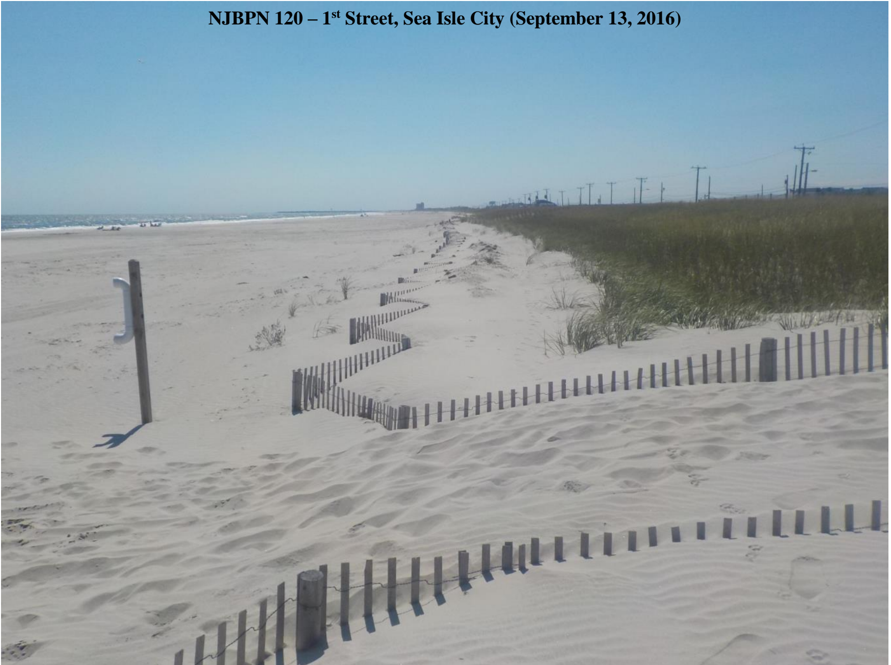
Figure 500. View to the south in the fall of 2016 showing sand accumulation at the fence line and the width of the dry beach.
