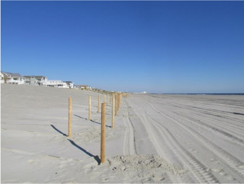
Figure 519a & 519b. The left photo was taken November 24, 2015 and shows the new fence line on the dune feature being installed during the federal project. The right photo, taken on September 12, 2016, shows the significant amount of wind-transported sand that was deposited around the newly installed, 4-foot high fence over a period of one year.
