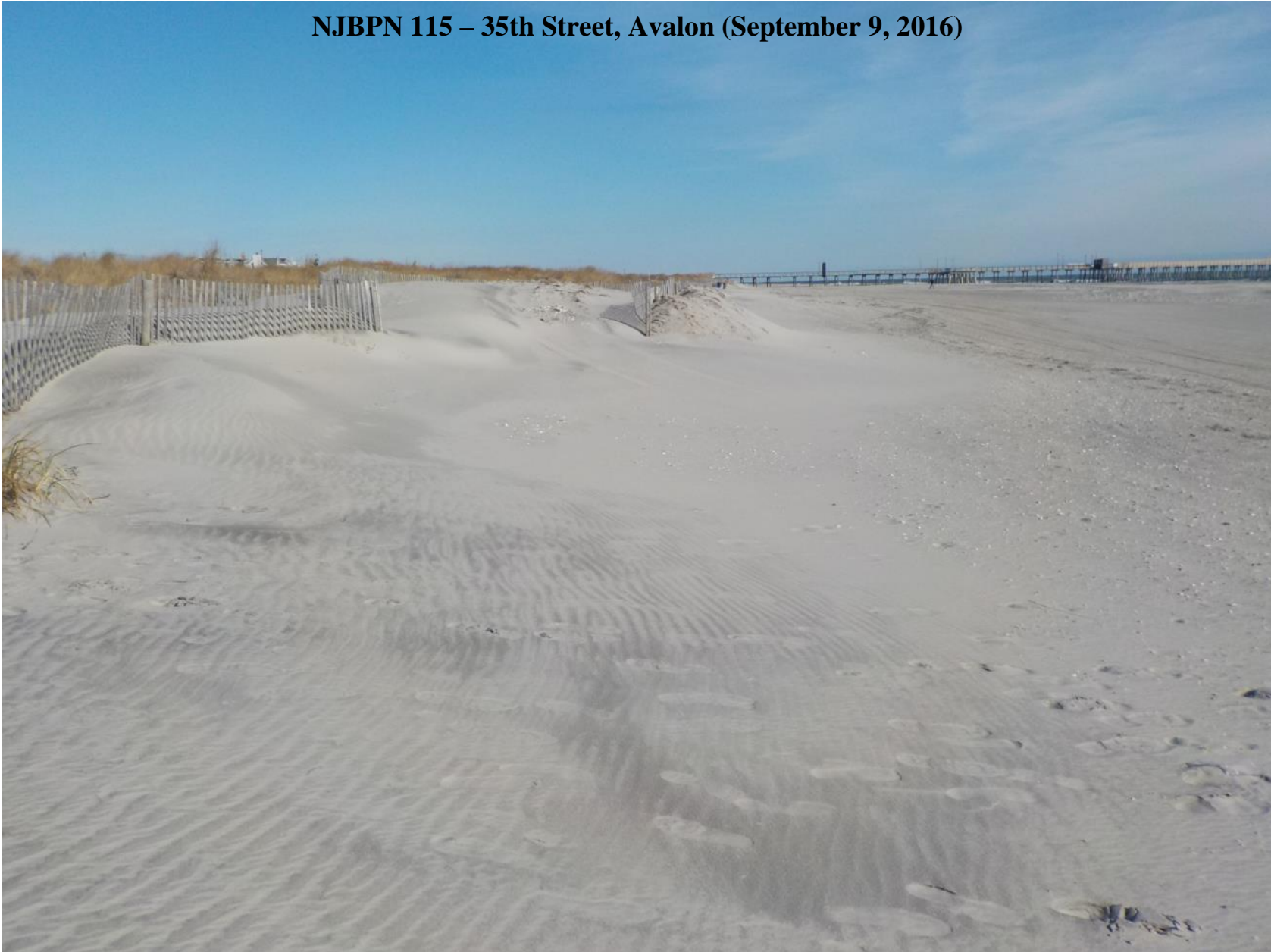
Figure 536. Looking north from the dune toe at 35 th Street in Avalon, the newly extended pier at 32 nd Street now reaches the ocean again. Sand was transported north from this site in 2016 by the Borough in a back-passing operation. Wind deposition has added to the dunes, while the harvest zone (for the back-passing operation) was completely filled back by June.
