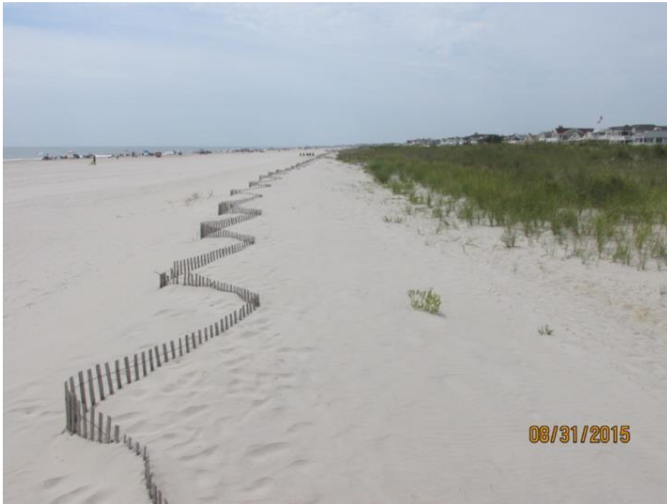
Figure 471a & 471b. The comparison photos show a view to the south (left taken August 31, 2015 and right photo taken September 16, 2016) and the extent of the beach at 34 th Street. The dune fencing has become almost buried from Aeolian transport and a large bar can be seen offshore in the photograph to the right.
