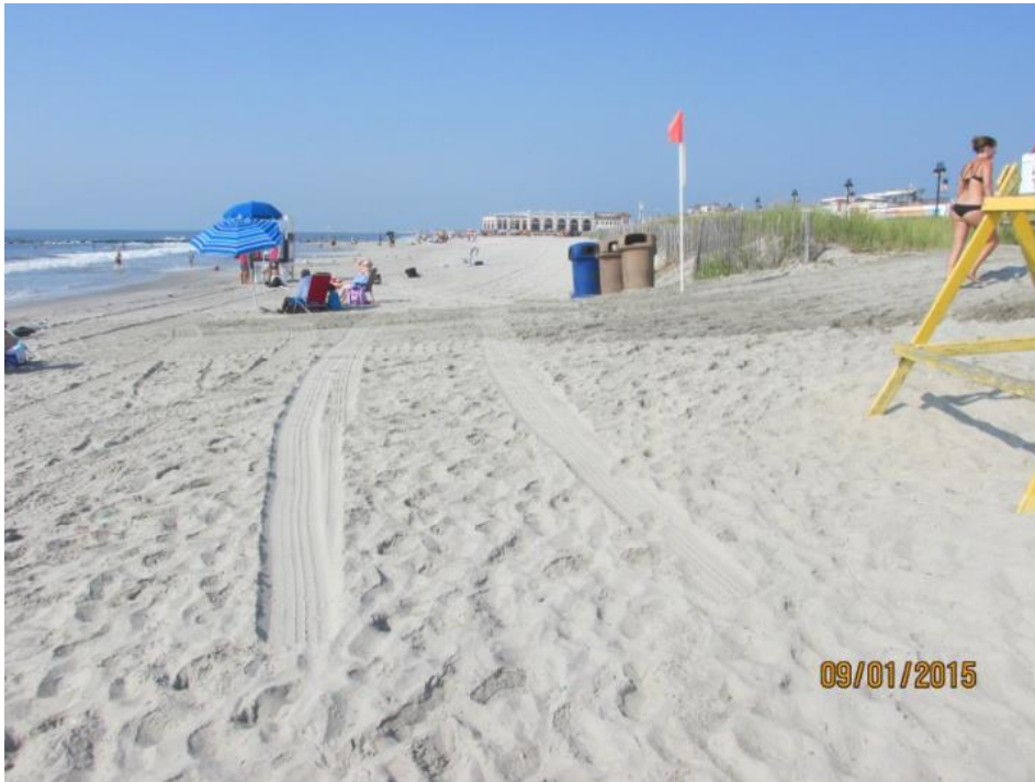
Figure 459a & 459b. The left photo (taken September 1, 2015) shows a modest berm still present from the USAACE (2013) beach fill. The right photo (taken September 20, 2016) shows approximately the same berm width with slightly more sand at the fencing.
