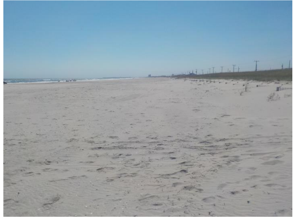
Figure 501a & 501b. Photo on the left was taken August 31, 2015 at the toe of the new foredune and the original dune that is located landward of the new fence was constructed in 1998 with a geo-tube core. The photo on the right was taken September 13, 2016, which was a year after the federal project. The dry beach width was increased and aeolian transport resulted in sand accumulating on the seaward dune slope.
