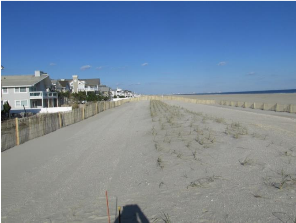
Figure 477a & 477b. In 2015, the 56 th Street site received its first sand replenishment since the 1995 state beach fill. The site is now included in the federally authorized project. The November 24, 2015 (left) photo shows the immediate post-project dune and berm. On the right (photo taken September 15, 2016) after a year of growth the grass appears healthy and vigorous. The wider beaches provide sand and space for continued natural dune development.
