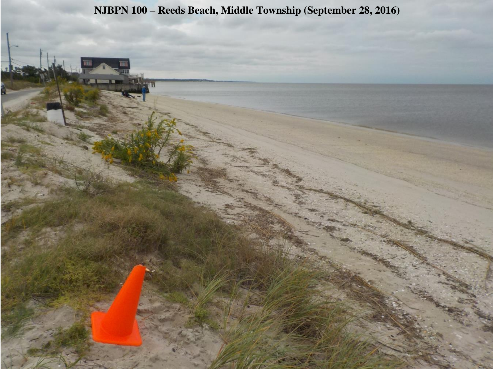
Figure 632. Reeds Beach is located on the northwest shoreline of Cape May County. The dune is small and maintained by removing sand from the road, while the beach is narrow and easily flooded in storms. Westerly wind-generated waves on Delaware Bay are particularly troublesome for this part of the county shoreline.
