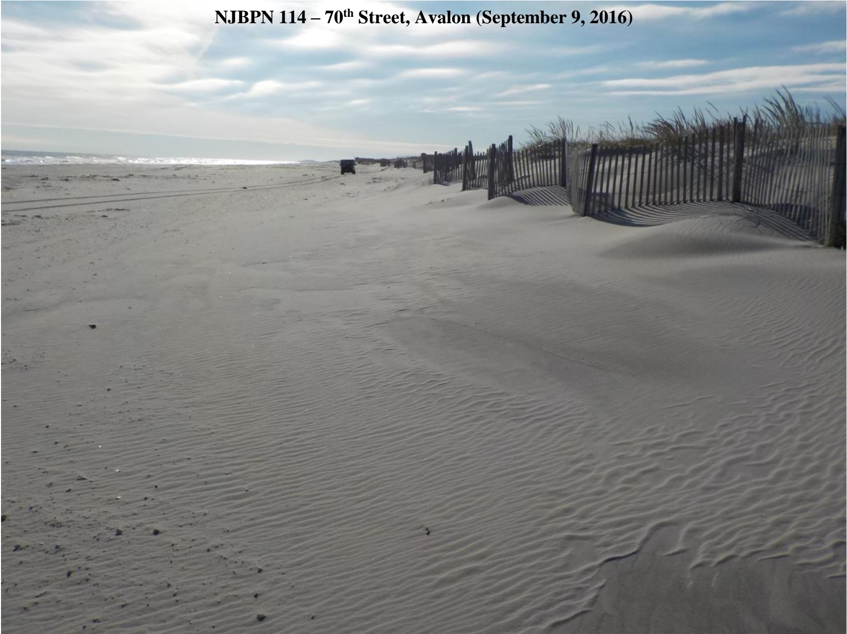
Figure 542. Looking south along the dune toe at 70 th Street in Avalon. This site is very stable, with the dune and beach accreting large amounts of sand. The accretional nature of this site is due to it being located at the northern taper of the federal project with sand only placed here once in 2003.
