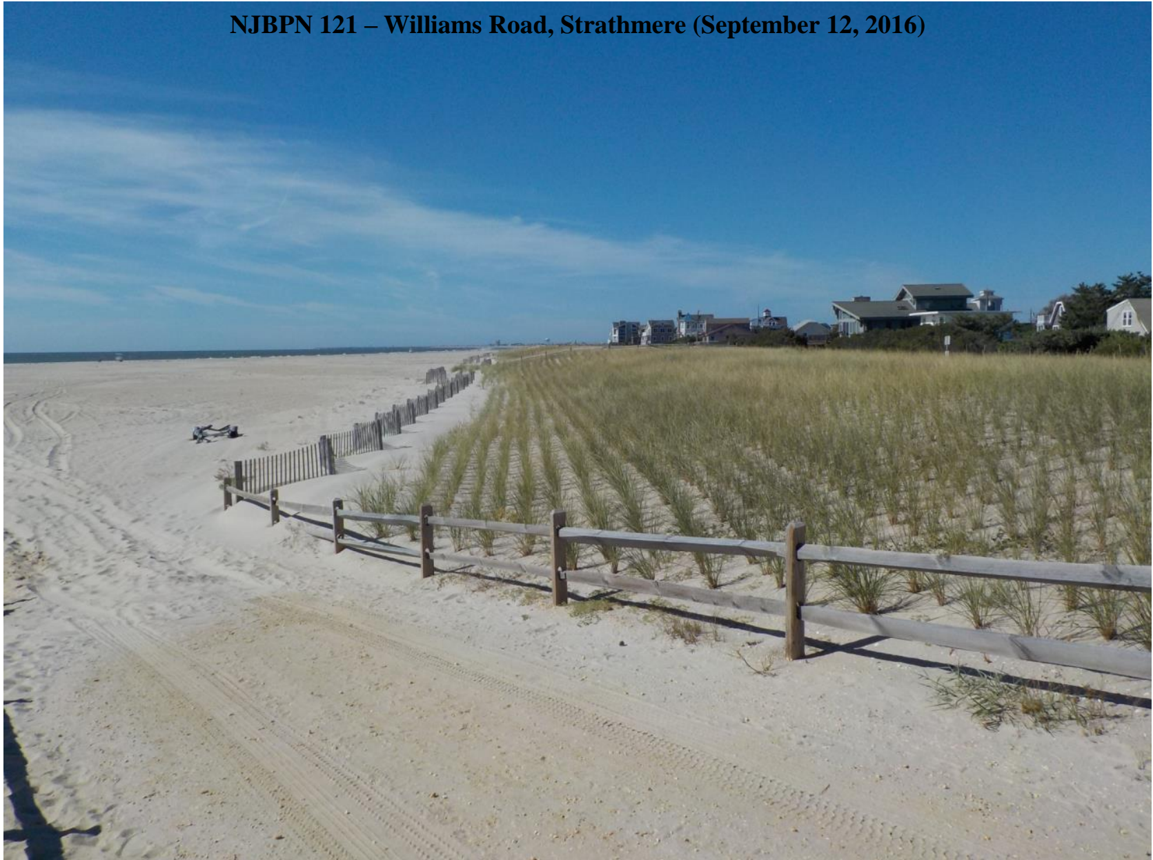
Figure 494. View to the south along the seaward dune toe from the vehicle access pathway to the beach. The plants are doing well and a small foredune is developing at the fence line.
