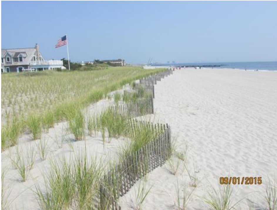
Figure 453a & 453b. The Gardens Road site is the northernmost profile in Ocean City and located in proximity Great Egg Inlet. (Left photo is from September 1, 2015. Right photo is from September 20, 2016). The dune and some of the berm that was created by the 2013 Federal emergency beach fill remained throughout 2015 and 2016. Seasonal berm elevation changes occurred, but the shoreline position was relatively constant. Over the 18-month study interval the site saw 25.21 yds 3 /ft in sand volume gains combined with a 28 ft shoreline advance.
