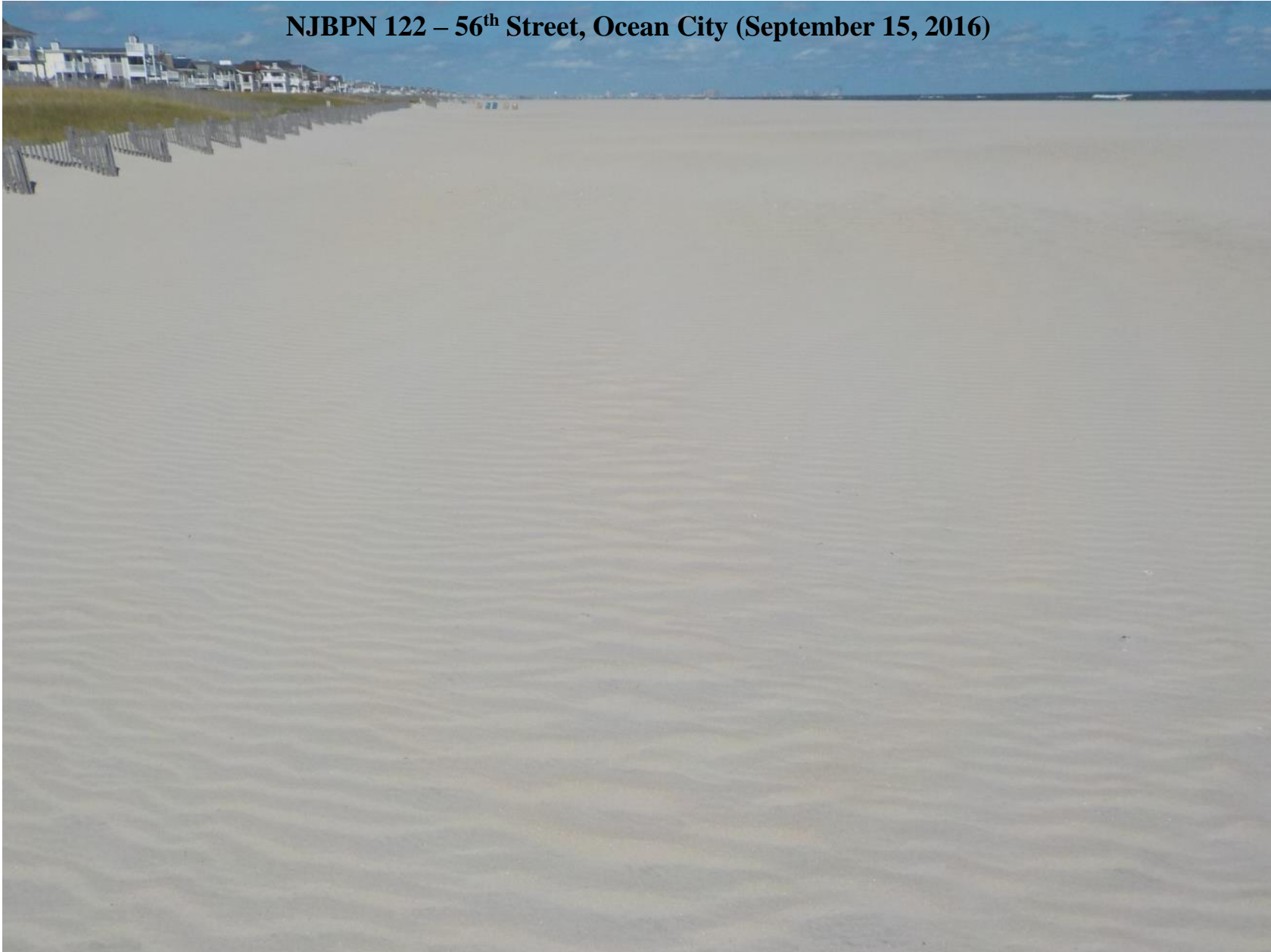
Figure 476. A view of the new federal beachfill looking north, with the dune grass in place and thriving. The width of dry beach is outstanding.
