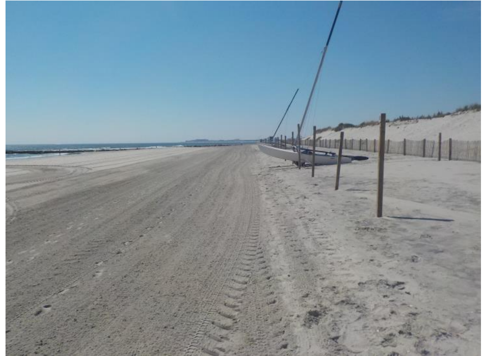
Figure 555a & 555b. The south end Stone Harbor site has shown a long-term erosional trend that may be influenced by changes surrounding Hereford Inlet. The site has been the recipient of numerous beach nourishment projects including municipal and Federal efforts. Most recent was spring 2013 as a post-Sandy restoration. The State of NJ is currently funding a maintenance effort into spring 2017. The left photo, taken on October 13, 2015, shows a wet beach nearly to the dune toe. By September 14, 2016 (right photo), the raked section of the beach was still subject to high tide wave run-up.
