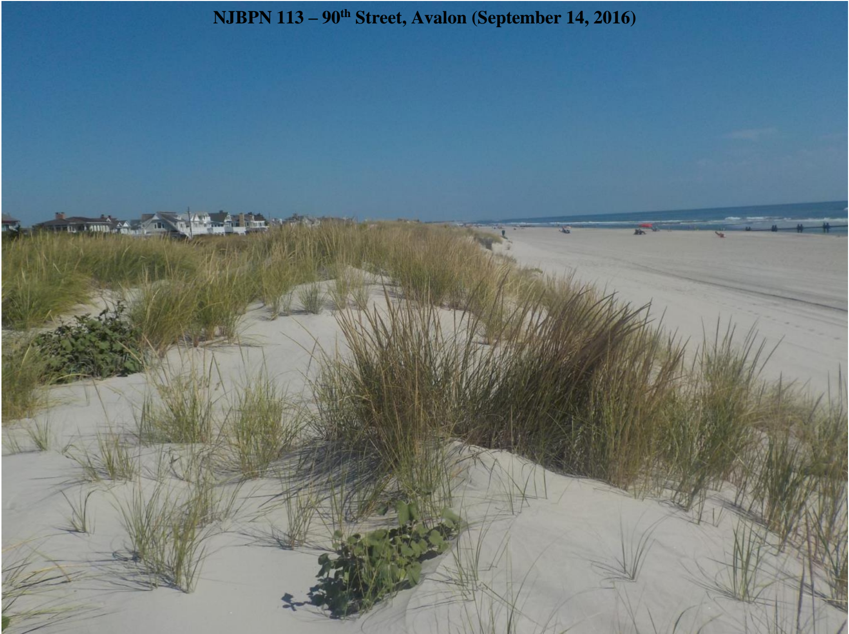
Figure 548. View north along the dune toe showing sand accumulation in the dunes and at the fence line. USACE work is anticipated here in spring 2017.
