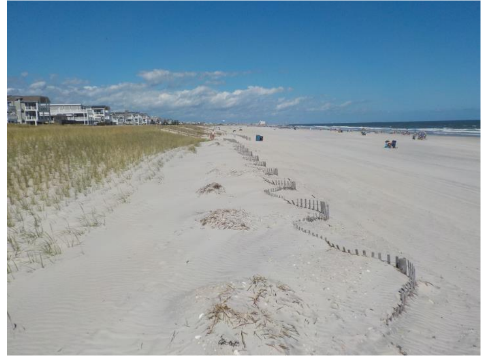
Figure 519a & 519b. The left photo was taken November 24, 2015 and shows the new fence line on the dune feature being installed during the federal project. The right photo, taken on September 12, 2016, shows the significant amount of wind-transported sand that was deposited around the newly installed, 4-foot high fence over a period of one year.
