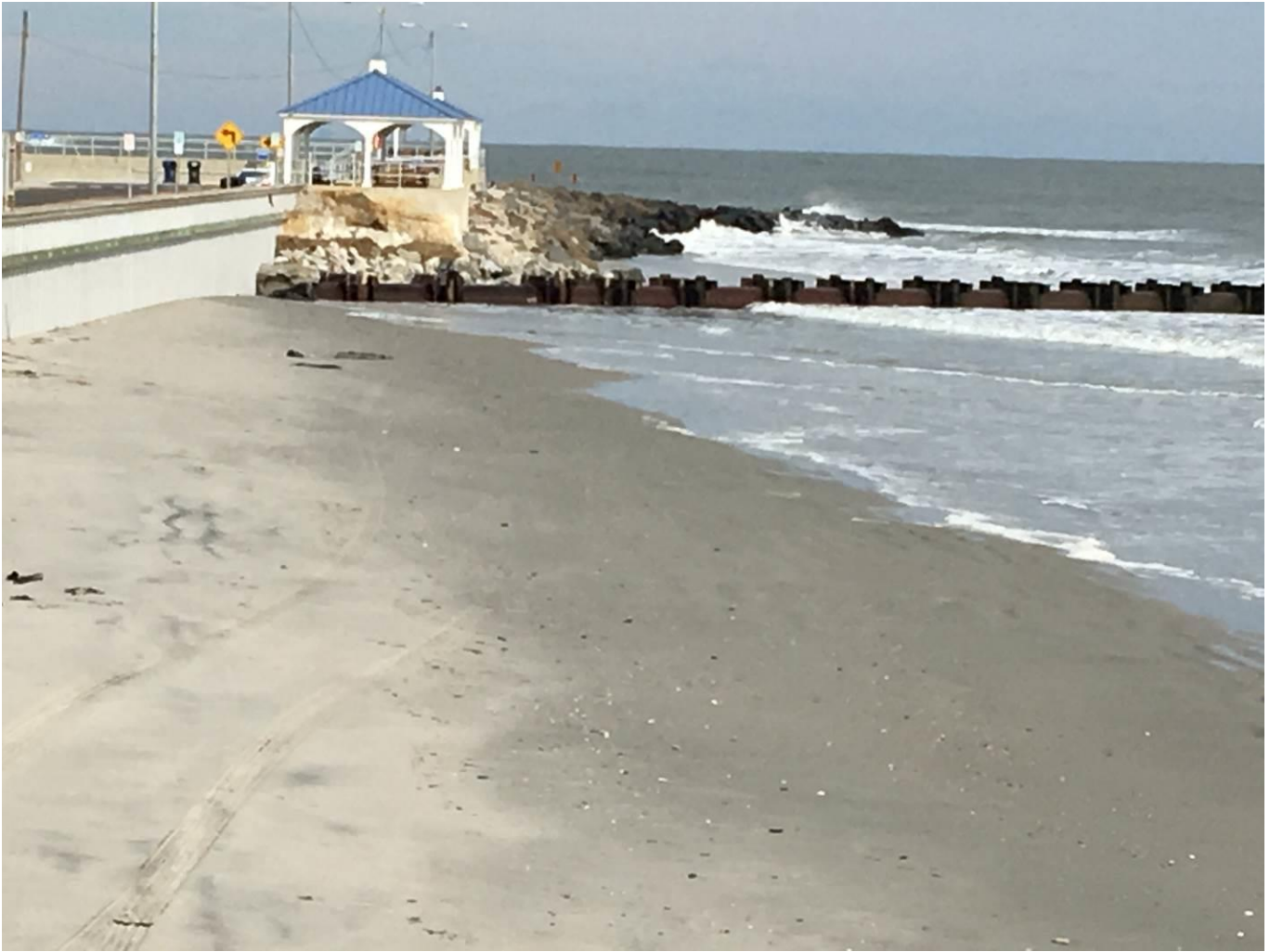
Figure 10. View to the north taken November 11, 2018 showing the inlet gazebo and inlet jetty beach. This position approximates 02+00 station with site 00+00 located on the other side of the pipeline.
