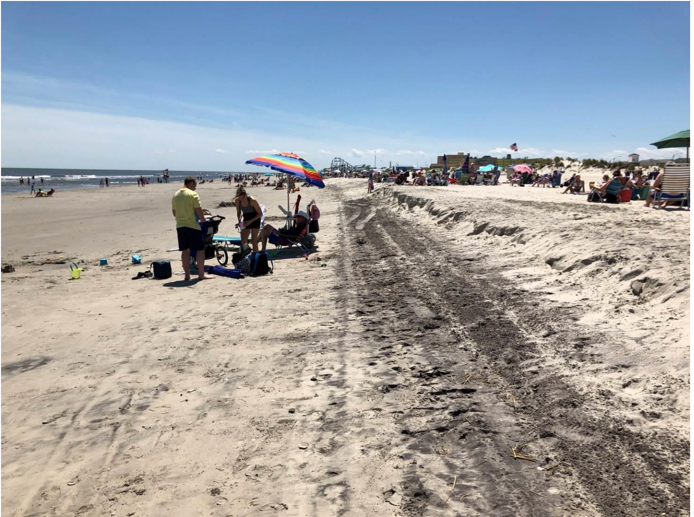
Figure 17. View to the south taken from the beach at 10 th Ave. on June 16, 2018 following sand placement from Wildwood. The erosion seen in the plot of surveys (Figure 14) is evidence that beach loss continued through the summer into the fall because the October 2018 survey plot shows a 67-foot shoreline retreat since the June 2018 survey. The annual retreat of 119 feet does show the storm impact during the spring of 2018.
