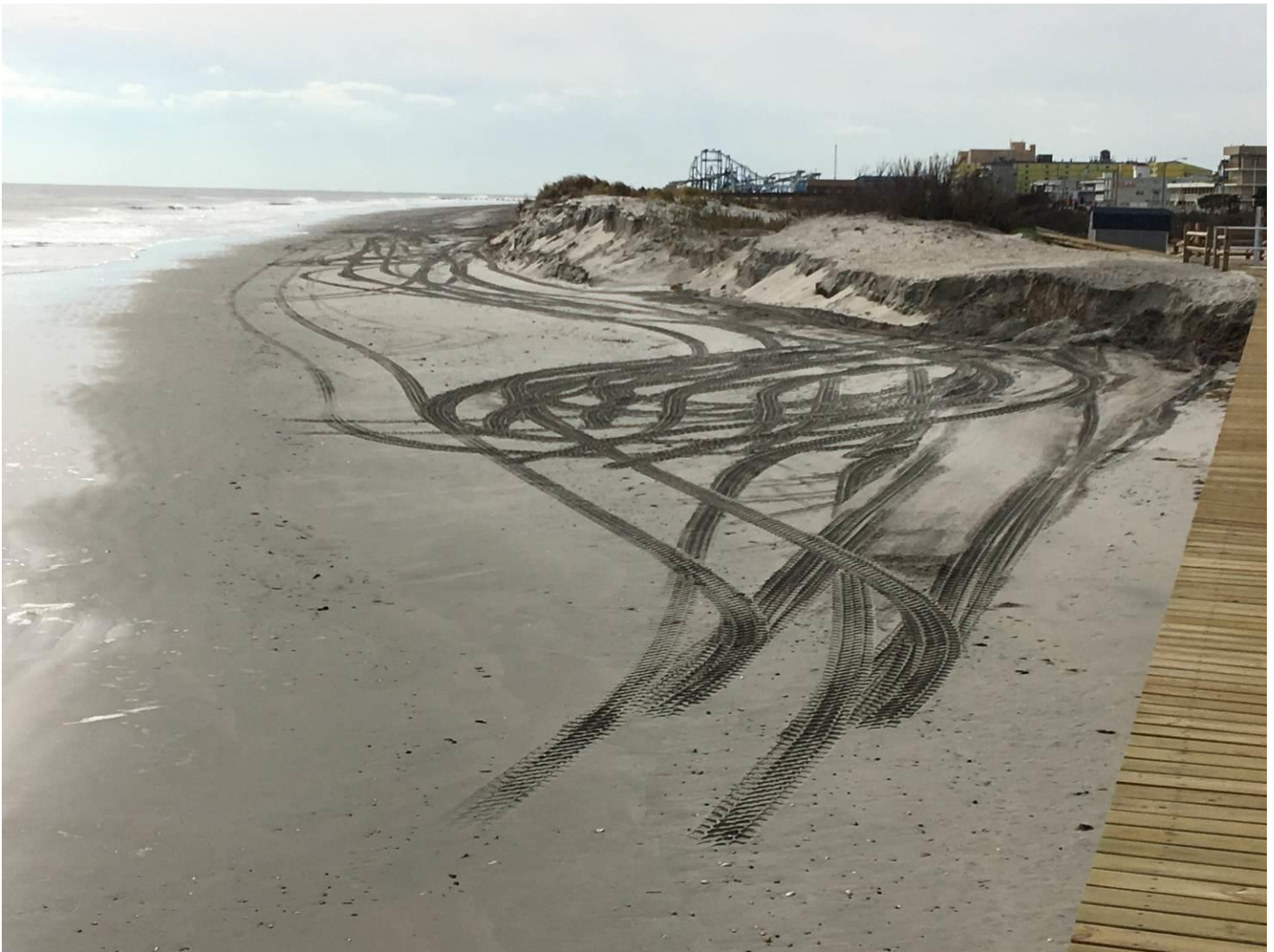
Figure 15. Site 06+00 is on the beach in proximity to where the dune returns to the beach. The view shows the extent of the erosion here and the minimal beach width remaining. The profile plot below paints a grim picture of dune loss and beach retreat reaching nearly 50 cubic yards of sand per foot since October 2017. In fact, the sand loss since June 2018 was 48.61 yds 3 /ft. meaning that it was the 2018 pattern of northeast storms from March into May that was responsible for the losses in spite of the sand transferred here from Wildwood by Memorial Day 2018.
