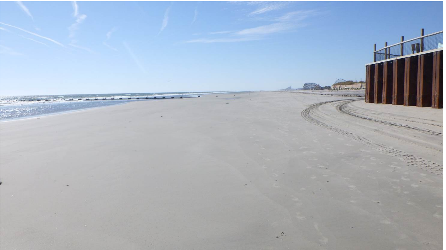
Figure 22. Transect 64+00 looking south into Wildwood City beaches shows that the beach width dramatically increases south of the Surfside Pier into Wildwood. Project maintenance efforts were dropped south to transect 73+00 following Hurricane Sandy and objections by Wildwood to managing the sand within the City limits.
