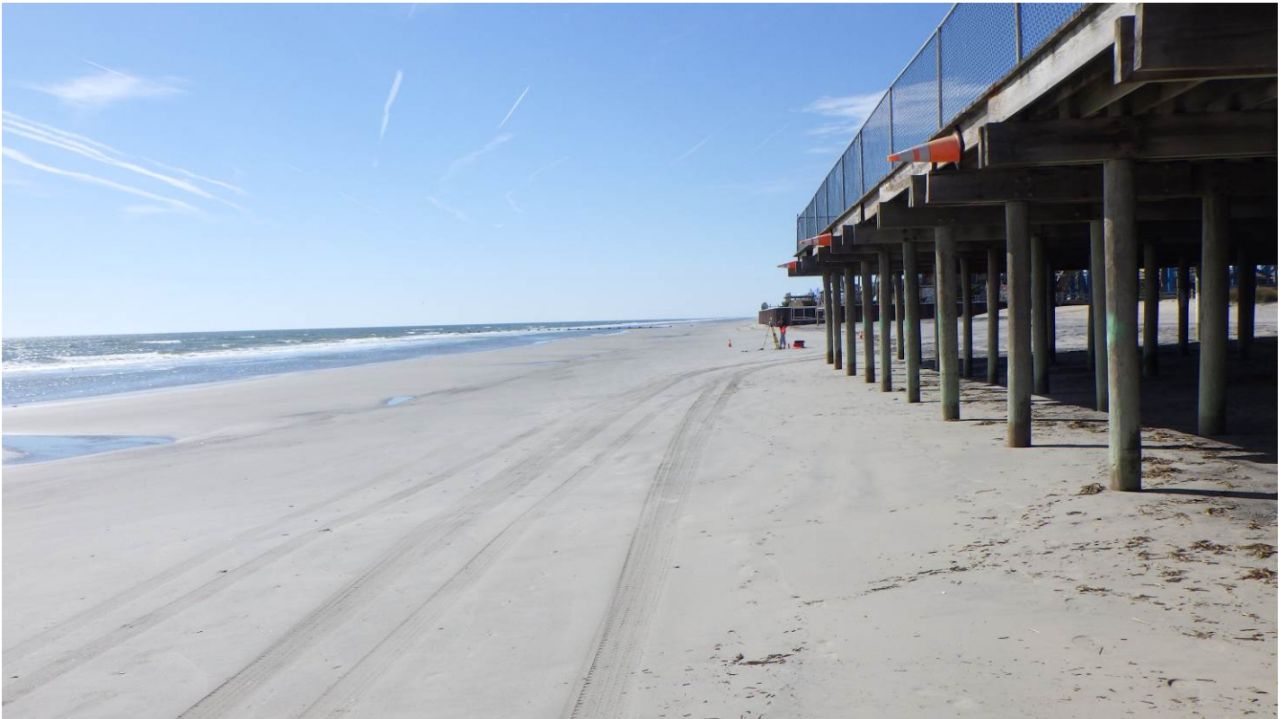
Figure 18. The June 16, 2021 view to the south looks across the front of the timber pier with the high tide line about 2 rows of pilings under the pier. The beach was wide and with a very low gradient which favors bathers but serves little in terms of storm protection.
