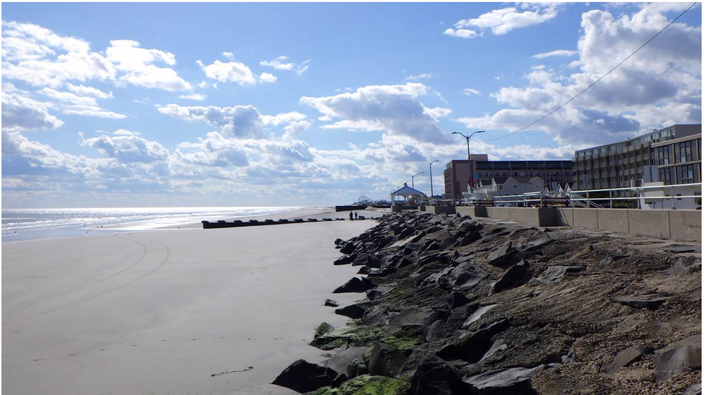
Figure 3. View to the south taken June 14, 2021 looking along the rock revetment past the 3 rd Ave. gazebo to the point where northerly transport has moved sand toward the jetty this past summer. The beach here has gained sand since mid-June 2021 both from the inlet ebb-tidal transport and littoral movement north from the graded-out stockpile. The rocks are still wet at high tide, but there is a wide, low gradient slope seaward into the offshore where most of the sand is deposited.
