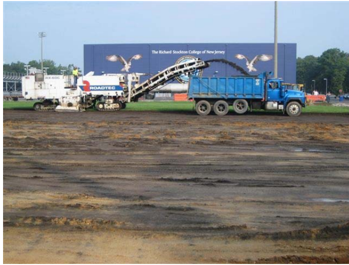
Photo: Stockton's 1.86-acre eco-friendly parking lot under construction.
