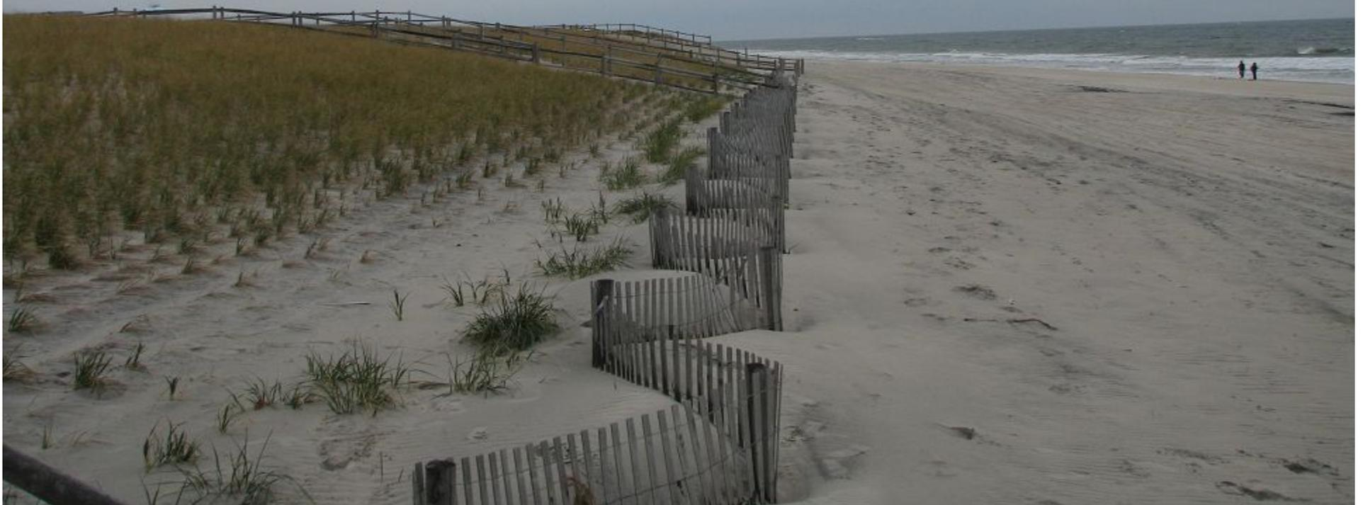
**Figure 222. Shown above is the view looking north from the fence line at Tranquility Drive in Harvey Cedars, NJ. The sand trapping effect of the dune fencing is apparent in this picture.**
