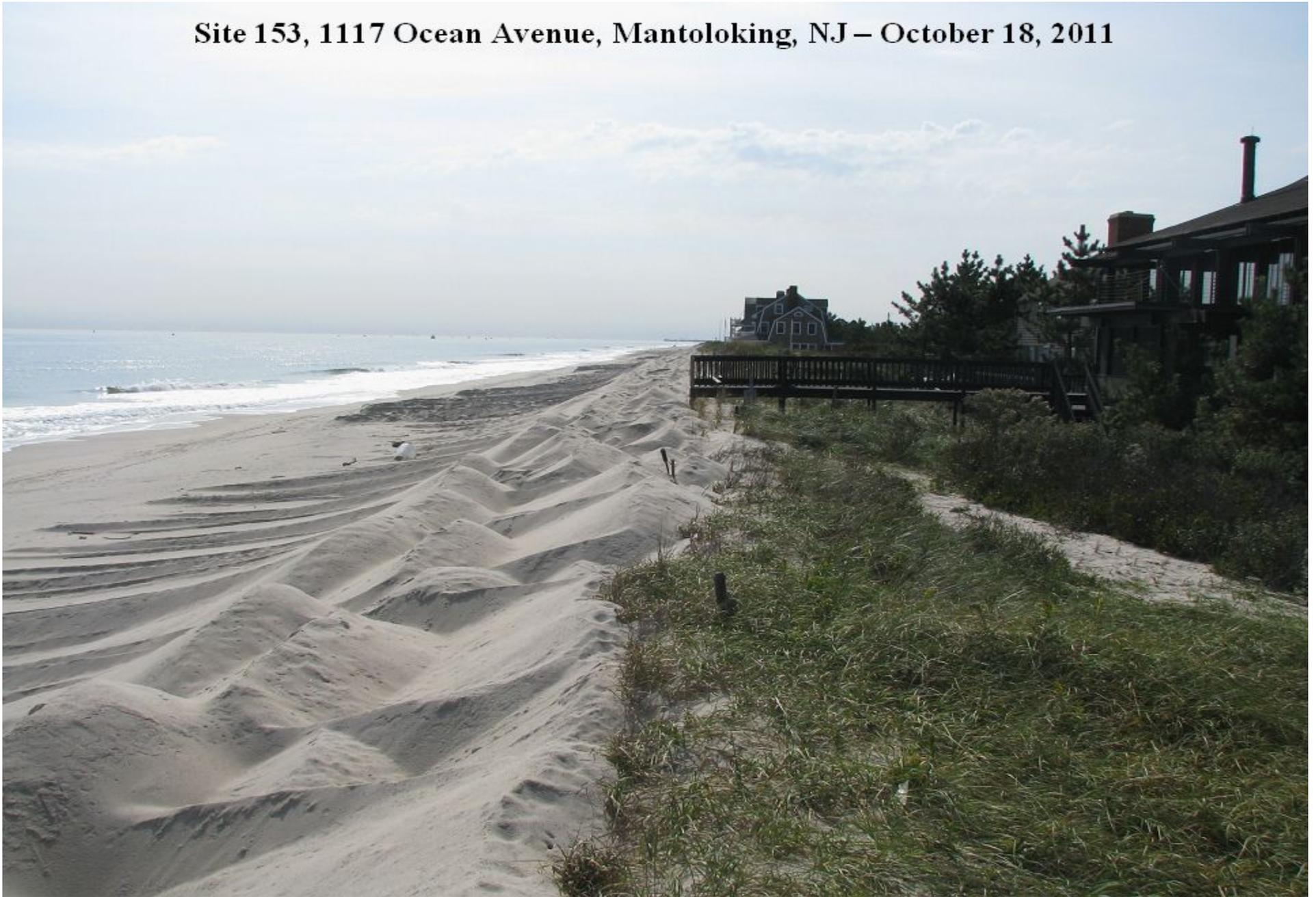
**Figure 163. Shown above is the view looking south from the dune crest at 1117 Ocean Avenue in Mantoloking, NJ. Bulldozing sand from the berm to the dune slope has become a common practice in the Borough of Mantoloking.**
