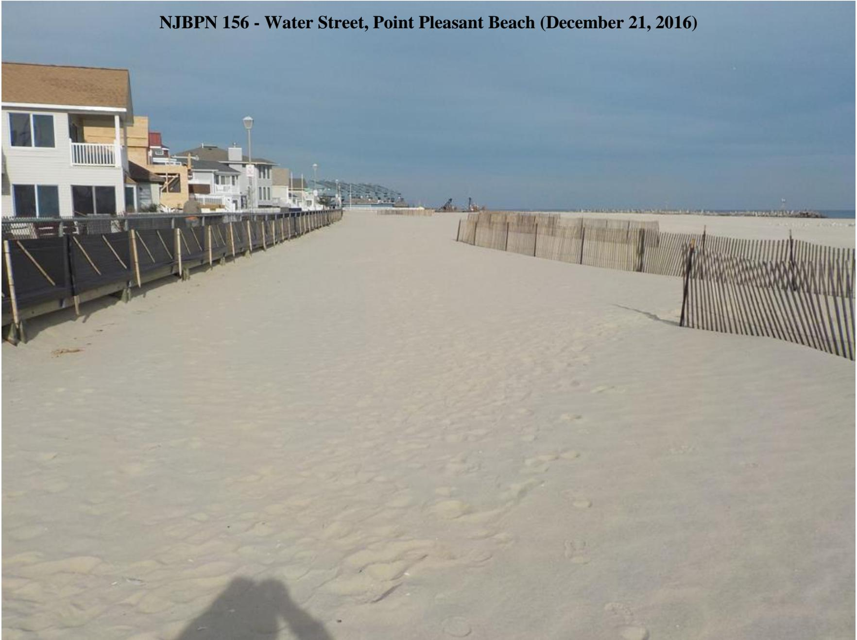
**Figure 219. View to the north from the backshore at Water Street in Point Pleasant Beach. The en eschelon rows of sand fence could be the locus of a dune along this section of beach. Any dune over 4 ft high would have prevented the overwash that was experienced during Hurricane Sandy.**
