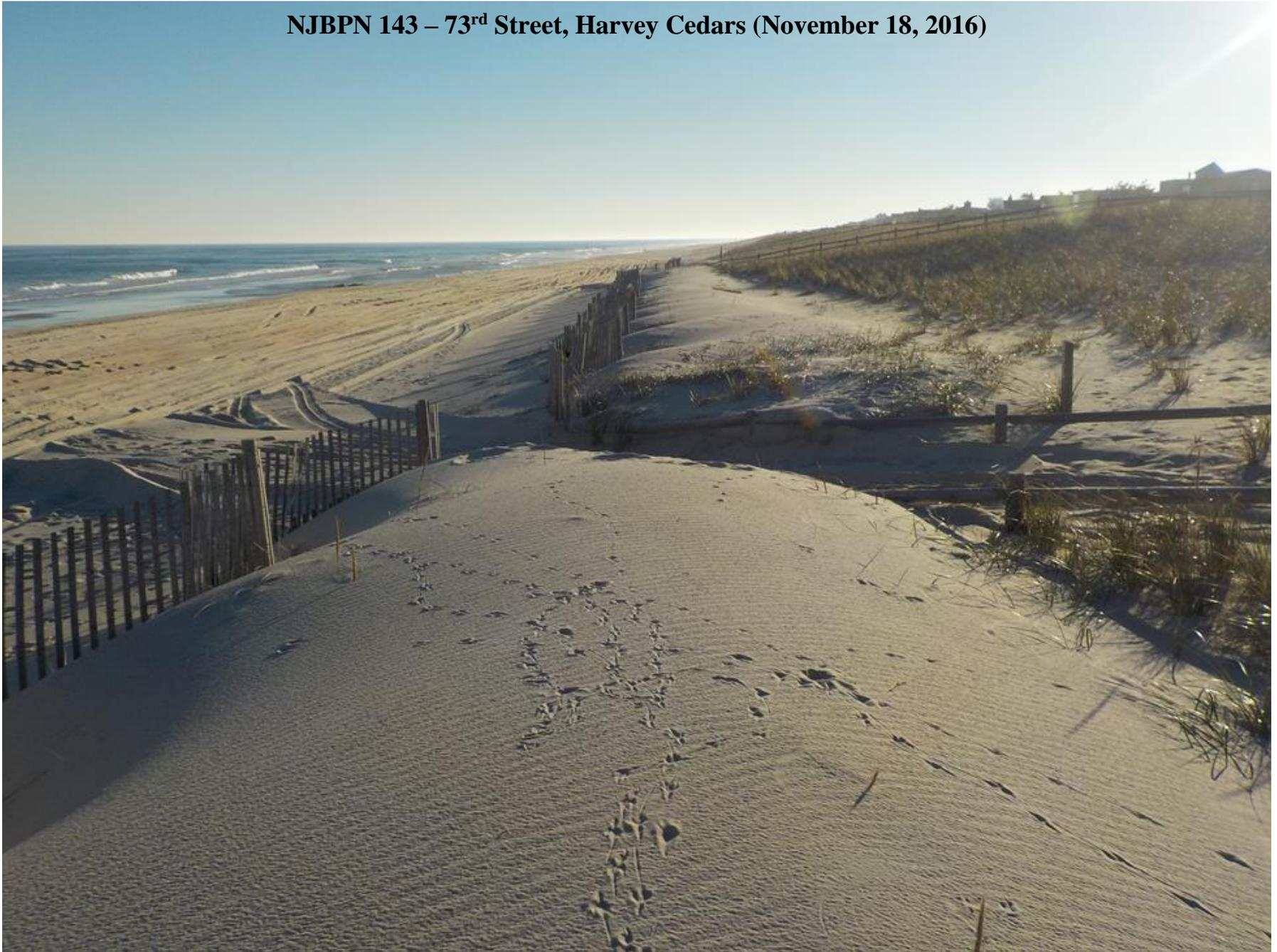
**Figure 322. View to the south from the dune at 73<sup>rd</sup> Street in Harvey Cedars. The accumulation of sand trapped by fencing adds to the dune's volume.**
