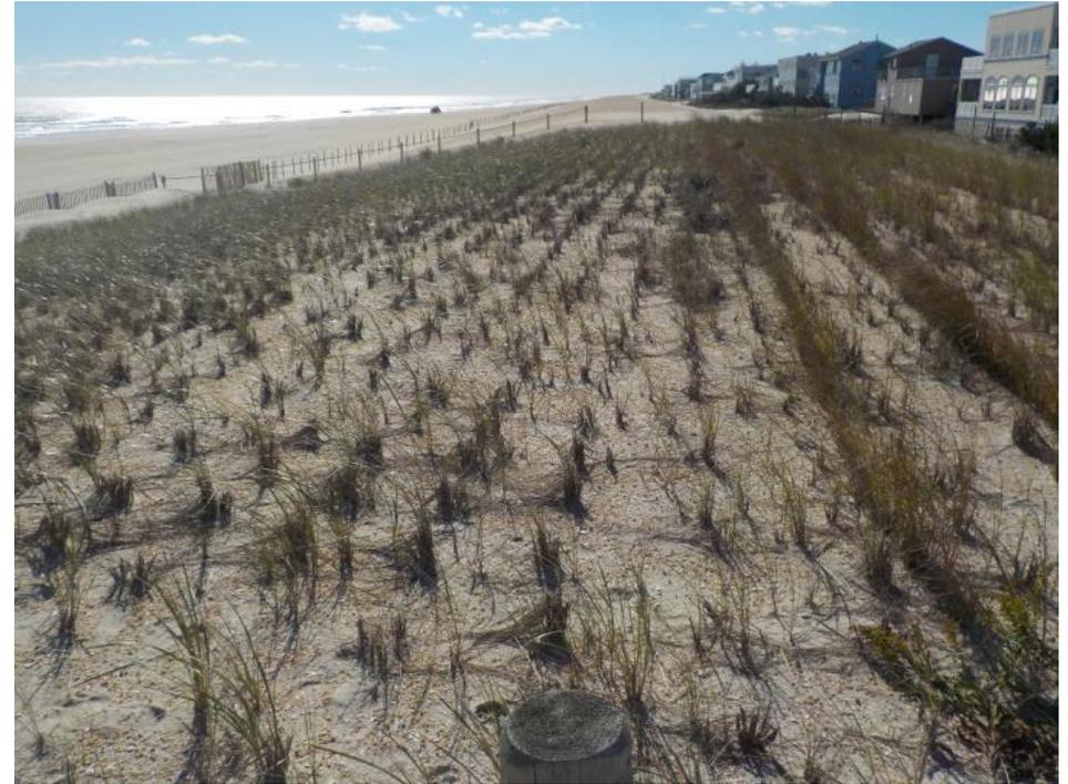
**Figure 329a & 329b. Conditions of the engineered dune have remained unchanged since the completion of the post-Sandy emergency beach fill. Sand accumulated at the seaward toe during fall 2016 (left taken September 16, 2015 and right taken October 28, 2016).**
