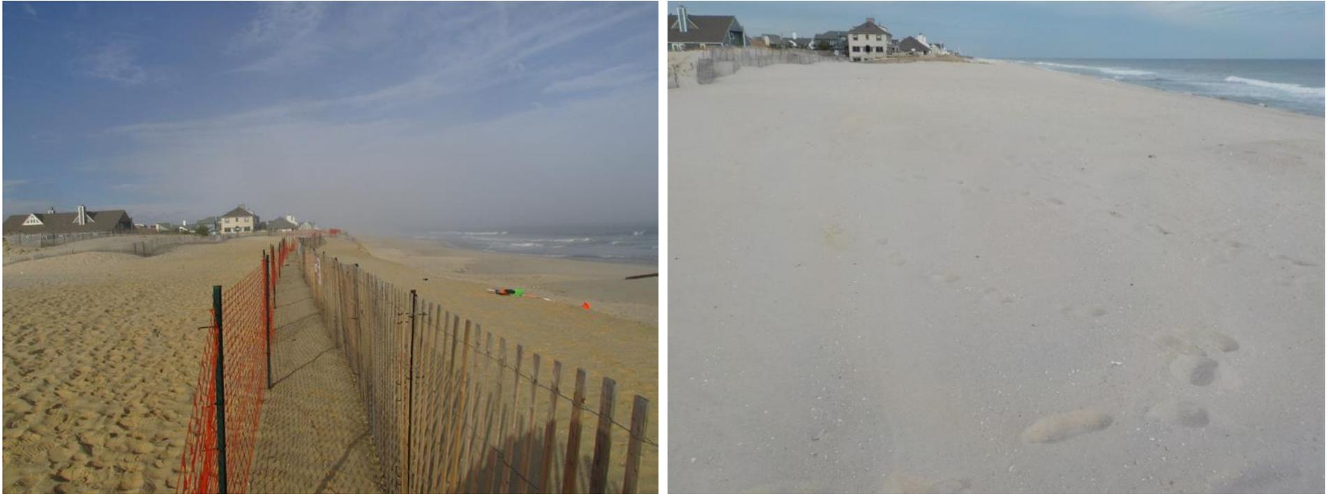
**Figure 245a & 245b. The view on the left was taken (December 14, 2015) with the new sand fence line erected along the sand ridge covering the steel bulkhead. Covered during the spring of 2016 following a northeast storm, the site returned to recreational uses by June 2016. The right photo was taken December 22, 2016 with a reasonable amount of beach width.**
