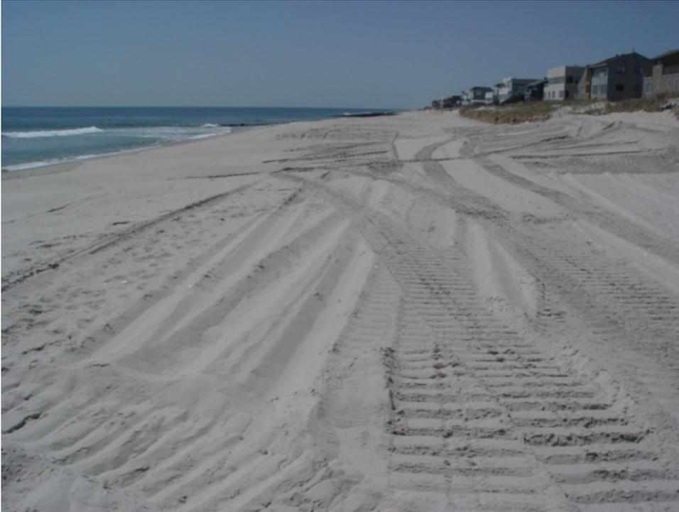
Figure 159. The beach at Tranquility Drive is narrow and the dunes are not sufficient to withstand moderate storm events. This April 20, 2006 photograph shows the beach following some municipal beach bulldozing to reinforce the dunes.
