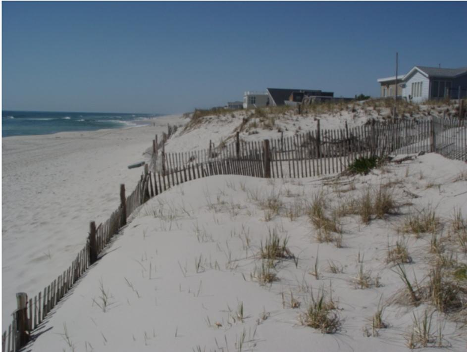
Figure 174. The dune at this site is higher and wider than some in other locations on Long Beach Island. The recent winter seasons have failed to reach the dune toe, which shows in the cross section plots. This photograph to the left was taken April 19, 2006 following the winter storm events.
