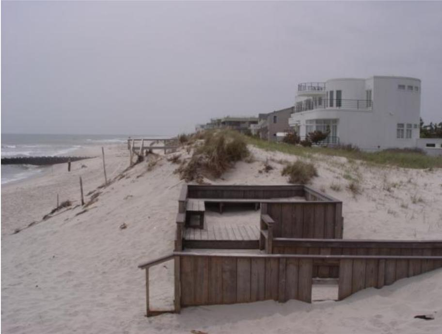
The dune in Loveladies is much narrower with the homes built into the landward toe so that any breach means that wave energy will accelerate landward into the buildings. This May 11th 2007 photograph shows a steep, narrow beach as well.
