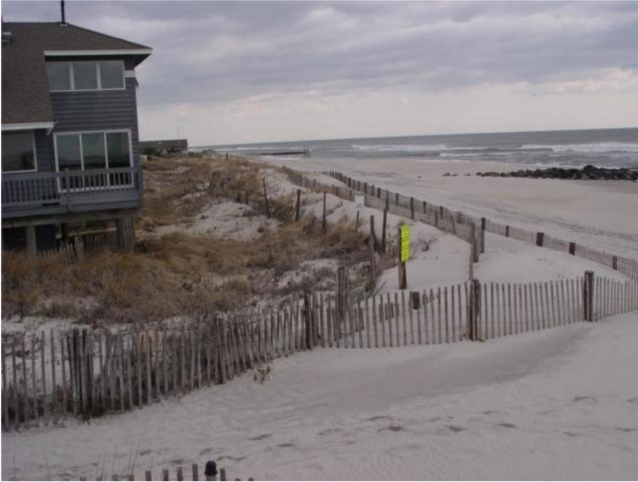
On April 13th 2007 the Dolphin Avenue site maintained a moderate-width beach with some growth in the dunes provided by three lines of fencing to trap sand. This situation is stable as long as moderate-intensity storm events do not occur.
