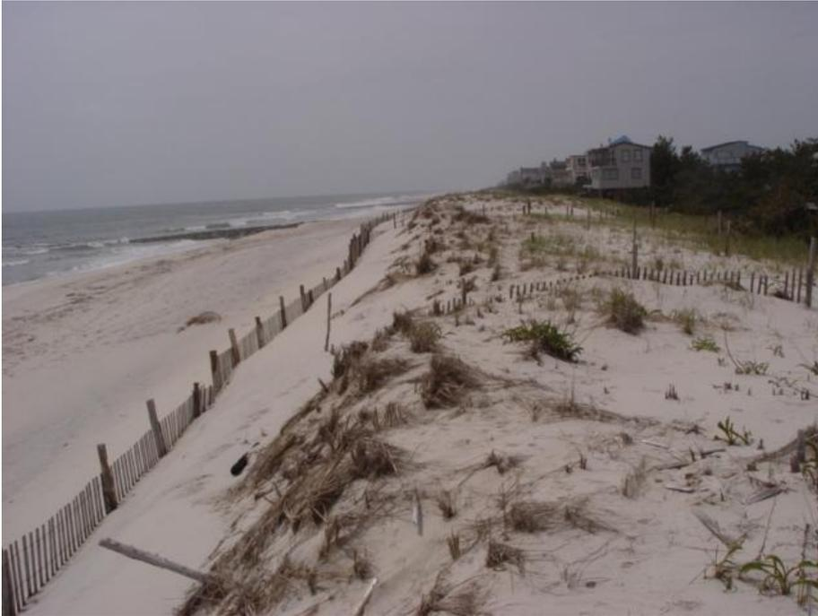
The northern Harvey Cedars site has a substantial dune and a moderately wide beach shown to the left on May 11th 2007. The dune crest vegetation is sparse, but the dune appears to have gained sand trapped at the straight fencing near the seaward toe.
