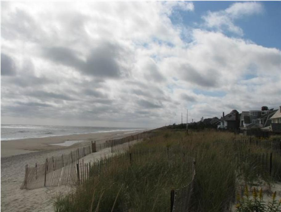
The October 14, 2008 photograph looking south shows a recently welded berm (note the incompletely filled pond in the middle ground along the back of the berm slope) and some additional grass growth over time. The site gained 14.11 yds<sup>3</sup>/ft. and the shoreline was 36 feet wider to the zero elevation position.
