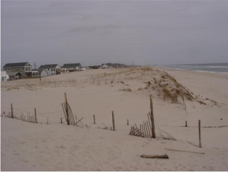
This site was moved south off the pedestrian pathway to allow the survey of the changes to the dune. When the site was established in 1986, there was no dune at all. By March 26th 2007 the accumulation of sand around fencing had produced a significant feature to increase the level of storm protection here.
