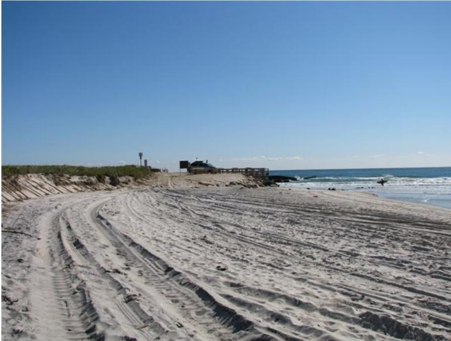
By October 7th 2008 sand has moved into the pocket between the groin and the profile line producing a 5-foot advance in the zero elevation position toward the ocean. The net sand volume was shifted offshore as the beach flattened (-13.08 yds<sup>3</sup>/ft.) and the offshore region gained 9.54 yds<sup>3</sup>/ft. The net change was a loss of 2.78 yds<sup>3</sup>/ft.
