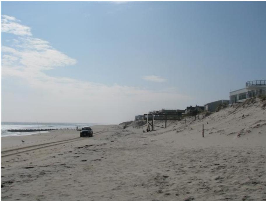
Changes by October 1st 2008 define a substantial summer berm in place between the vehicle in the photograph and the shoreline. The berm represents a gain of 21.06 yds<sup>3</sup>/ft. between the beach (+8.28 foot elevation) and the offshore (-5.40 feet). Loss further seaward reduced the gain to 7.12 yds<sup>3</sup>/ft. combined with a shoreline advance of 31 feet. This change is typical of summer accretion along the Long Beach Island coast.
