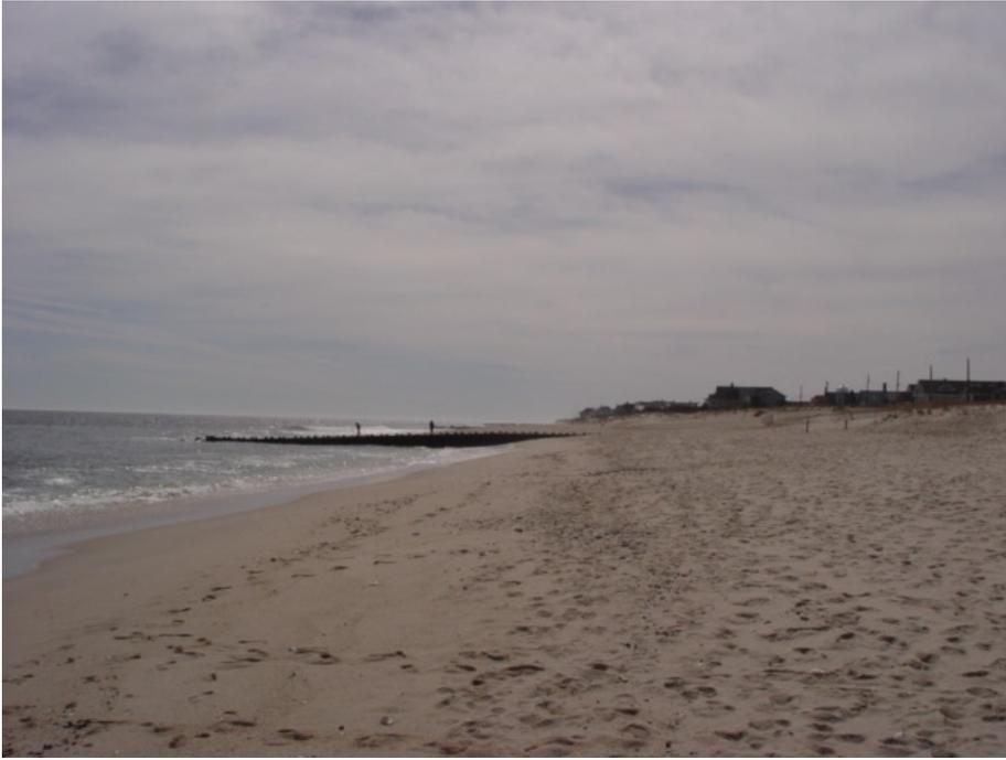
This view to the south on March 12th 2007 shows the first groin in Bay Head producing a significant offset to the south. This is common when waves move sand toward the north along this beach segment.
