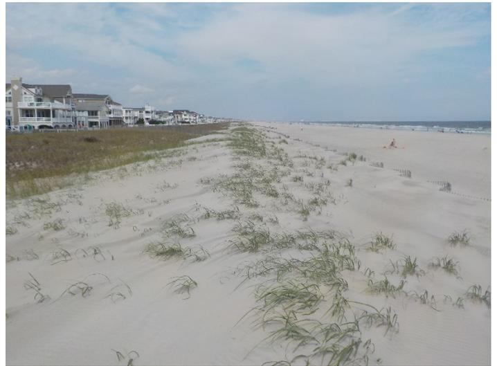
In 2015, the 56<sup>th</sup> Street site received its first sand replenishment since the 1995 state beach fill. The new dune was planted and fenced as shown on the left photograph (September 22, 2017). The right view was taken September 18, 2018 and shows that the newest line of sand fencing has been completely buried by Sept. 2018.
