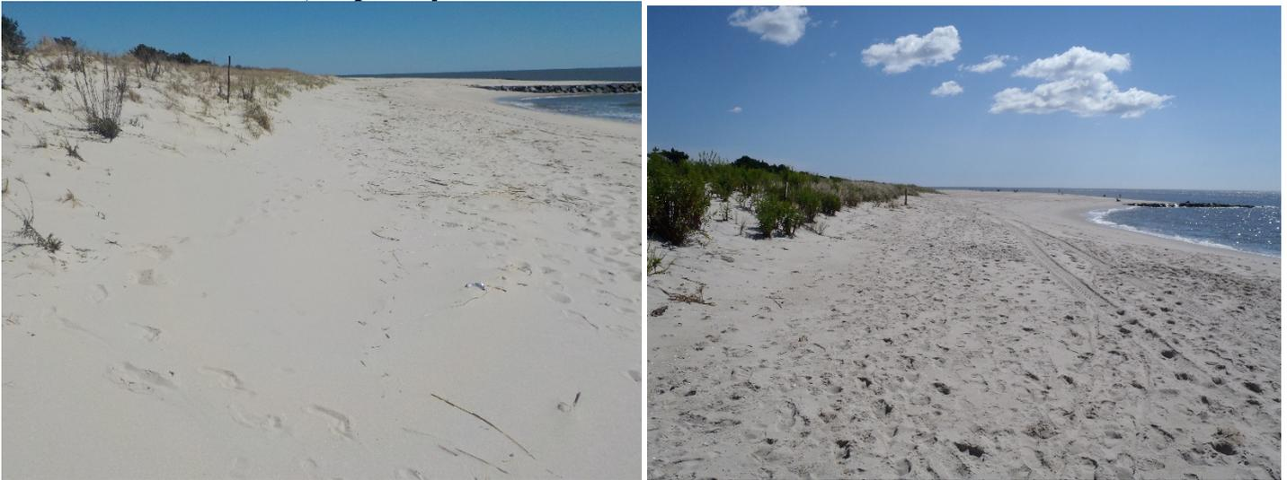
The left photo was taken on April 20, 2016. The right photo was taken on September 21, 2017. Sand was added by the USACE as far west as this groin cell in Cape May Point by spring 2017 with loss in beach width subsequently.
