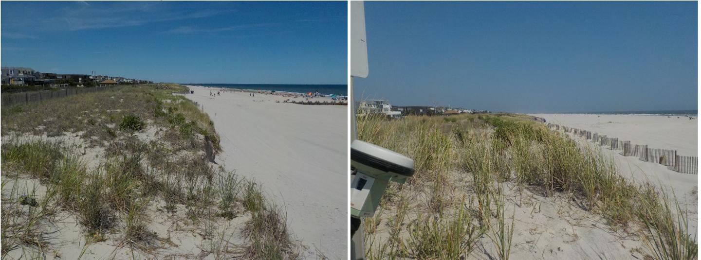
The left photo (taken June 14, 2016) shows a reduced-width dry beach following the loss of Borough-funded fill effort in 2015. The right photo taken on September 8, 2017 following the most recent federal maintenance. The new fencing has already gained some sand at its base.
