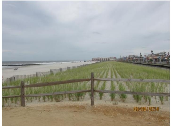
The October 16, 2013 view shows (left), the berm and dunes restored to design elevation by the ACOE. Beach volume loss has reduced the beach width, but the dunes and the new grass plants are doing well as of September 8, 2014.
