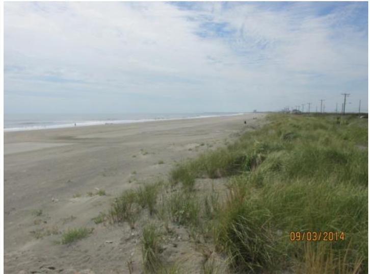
The dune here at the 1<sup>st</sup> Street location consists of a geotextile core covered by sand. Storm damage was minimal and natural recovery has blended in well with the surviving vegetation. The majority of the accumulation has been in the form of a wider beach and much larger summer berm. Sand moved onto the shoreline from bars built offshore.
