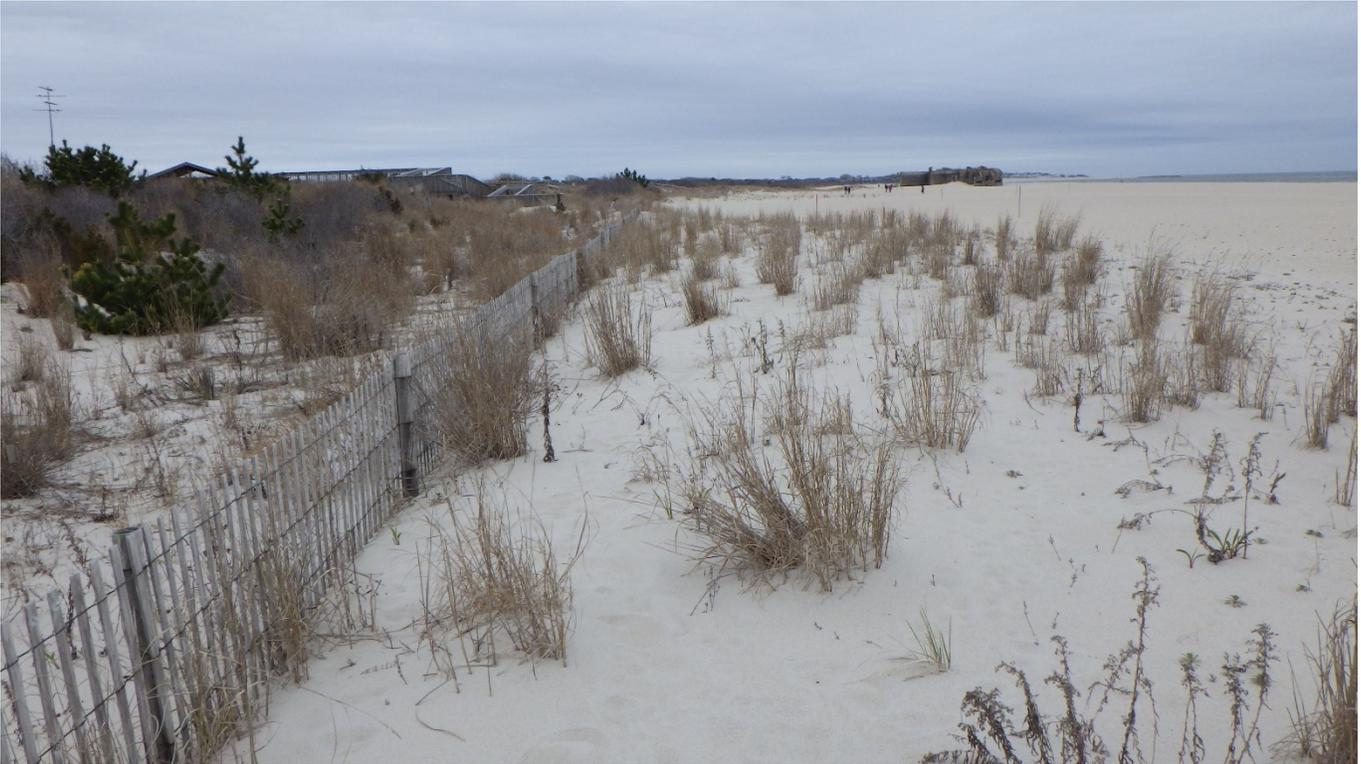
***Figure 2. The view was taken April 9, 2021 showing the transition into the NJ State Park and with Cape May City in the far distance. This view is from the seaward toe of the dunes where grass has grown seaward beyond the fence. Prior to this project the concrete WW II control bunker was entirely in the ocean.***
