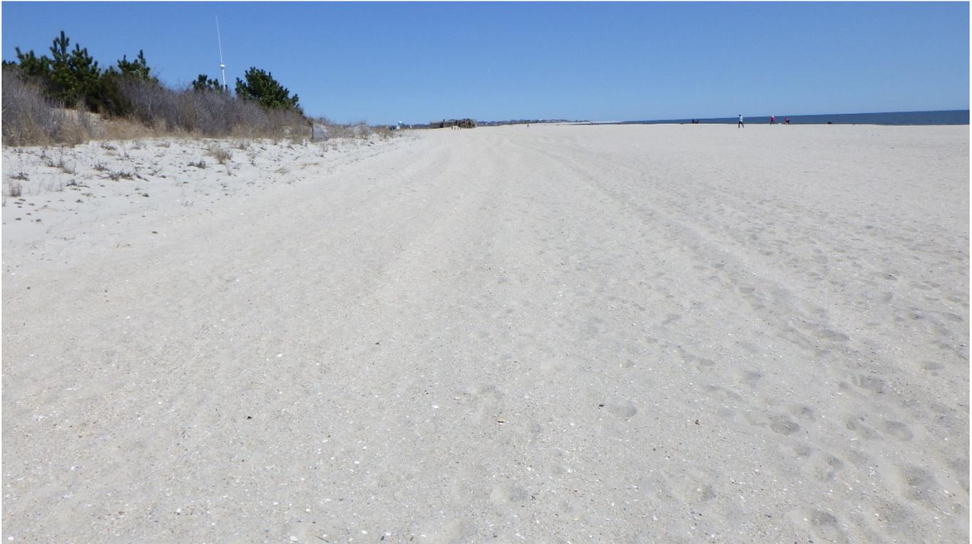
*Figure 4. This view is to the northeast showing the beach width present as of April 8, 2021. The dune to the left side sits on top of the stone revetment and the beach is many times the pre-beach nourishment width creating an excellent storm barrier as well as a recreational resource enjoyed by the Borough citizens.*
